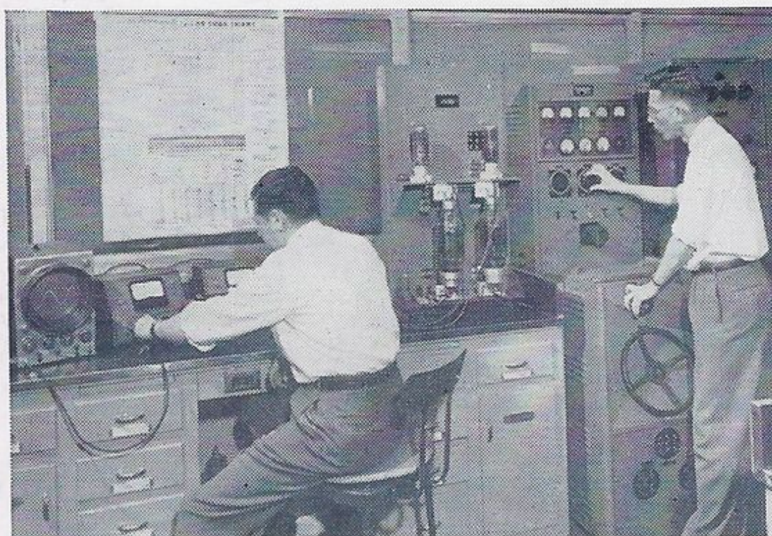
Testing modulation transformer under operating conditions
